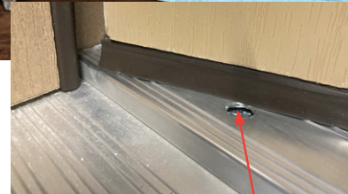
ADJUSTABLE SCREWS (WEATHER SEAL IS HIDDEN FOR ISCS)
