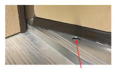
ADJUSTABLE SCREWS (WEATHER SEAL IS HIDDEN FOR ISCS)
