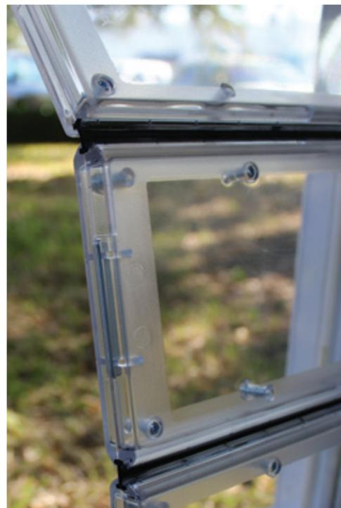
The flexible LEXAN flap uses durable vinyl weatherstrip and rare earth magnets to create an energy efficient seal when not in use.
