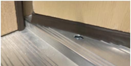
Inswing or outswing threshold mill finish
